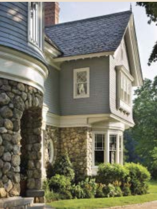
15,000 sf | round fieldstone facade with bluestone accents, including patio and steps
